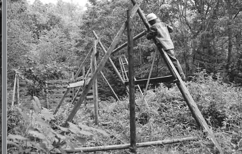
▲防鹿柵の補修
